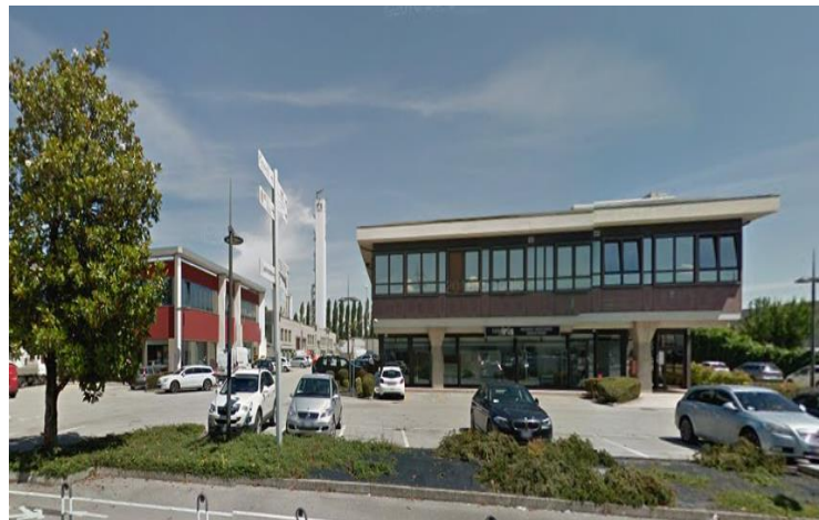
IRS offices @ AT Invest innovation center Padova
